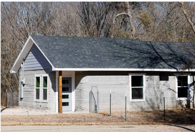
MRB Robotics has now built two three-bedroom homes in Mabank using a 3D printer. (Shafkat Anowar / Staff Photographer)
